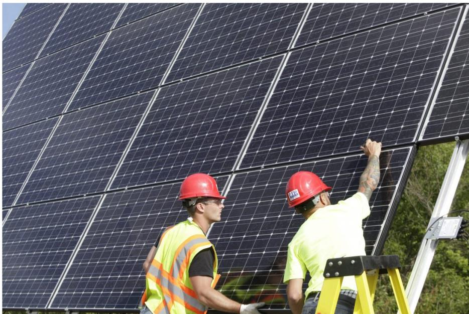
*Edward Sarcione, left, and electrician Joe Kilijanski of CIR Electrical Construction Corp. install an array of solar panels made by Silevo on a “tracker” system that automatically follows the sun to optimize the system’s performance at a residence in Marilla, Friday, June 20, 2014. (Derek Gee/Buffalo News)*
