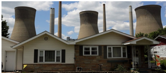
The John Amos coal-fired power plant is seen behind a home in Poca, West Virginia, in 2014. (photo: Robert Galbraith/Reuters)
